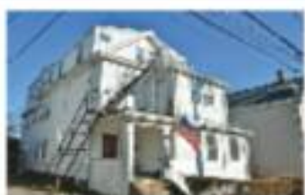
Salemville 5 Family $ 999,900 면적 $ 7000, 주거 면적 3072 sq. ft. 2차 주택기 501 콘크리트, Quaker 4 Doors, Hard oak floor, porcelain granite, stainless steel hood, Central Air Conditioning, and in-law bedroom, 2nd floor 4th flr.
