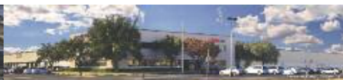
Texas, USA Plant
